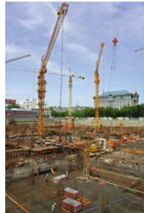
Retail space construction, Beijing. by Daniel Allen
